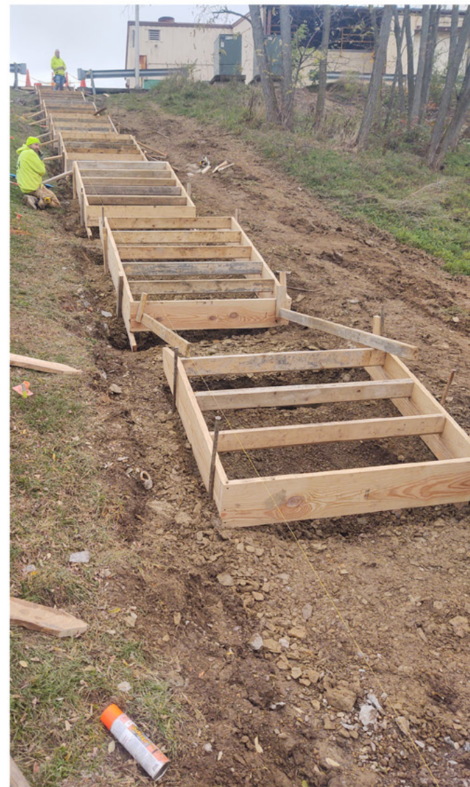
Top: A look from the top of the stairwell during demolition. Middle: The new concrete steps forms being built. Bottom: Contractors are pouring concrete into the new stair forms. U.S. Air National Guard photos by: Tech. Sgt. Jason Nelson
