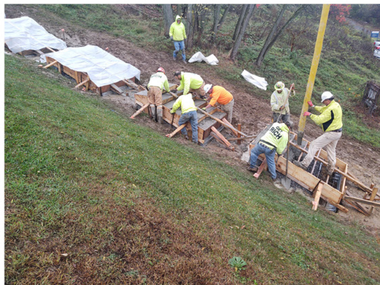
Top: A look from the top of the stairwell during demolition. Middle: The new concrete steps forms being built. Bottom: Contractors are pouring concrete into the new stair forms. U.S. Air National Guard photos by: Tech. Sgt. Jason Nelson
